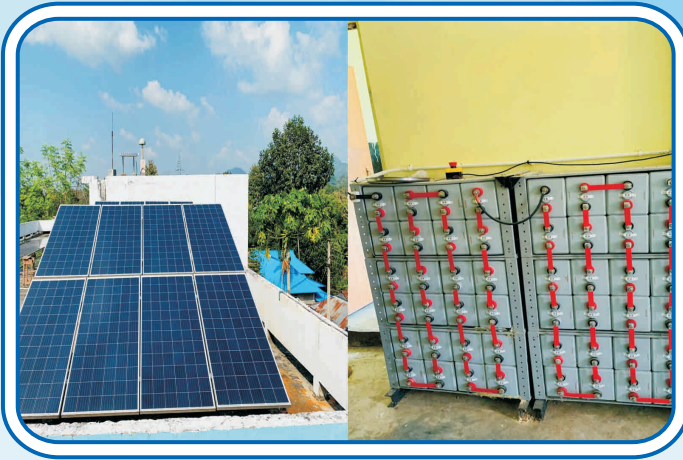
Installation of Solar Hybrid Power Plant in Tripura
