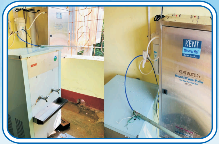
Installation of Solar RO Plant in Tripura
